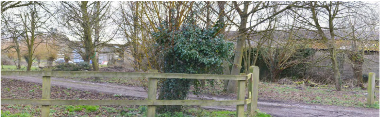
Photo 3: View from north-west on Caps Lane showing barns and line of willow
